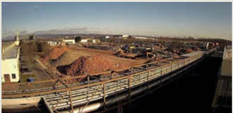
Demolition works at brownfield VGP Park Wiesloch-Walldorf with recyclable materials and soil being sorted and separated
